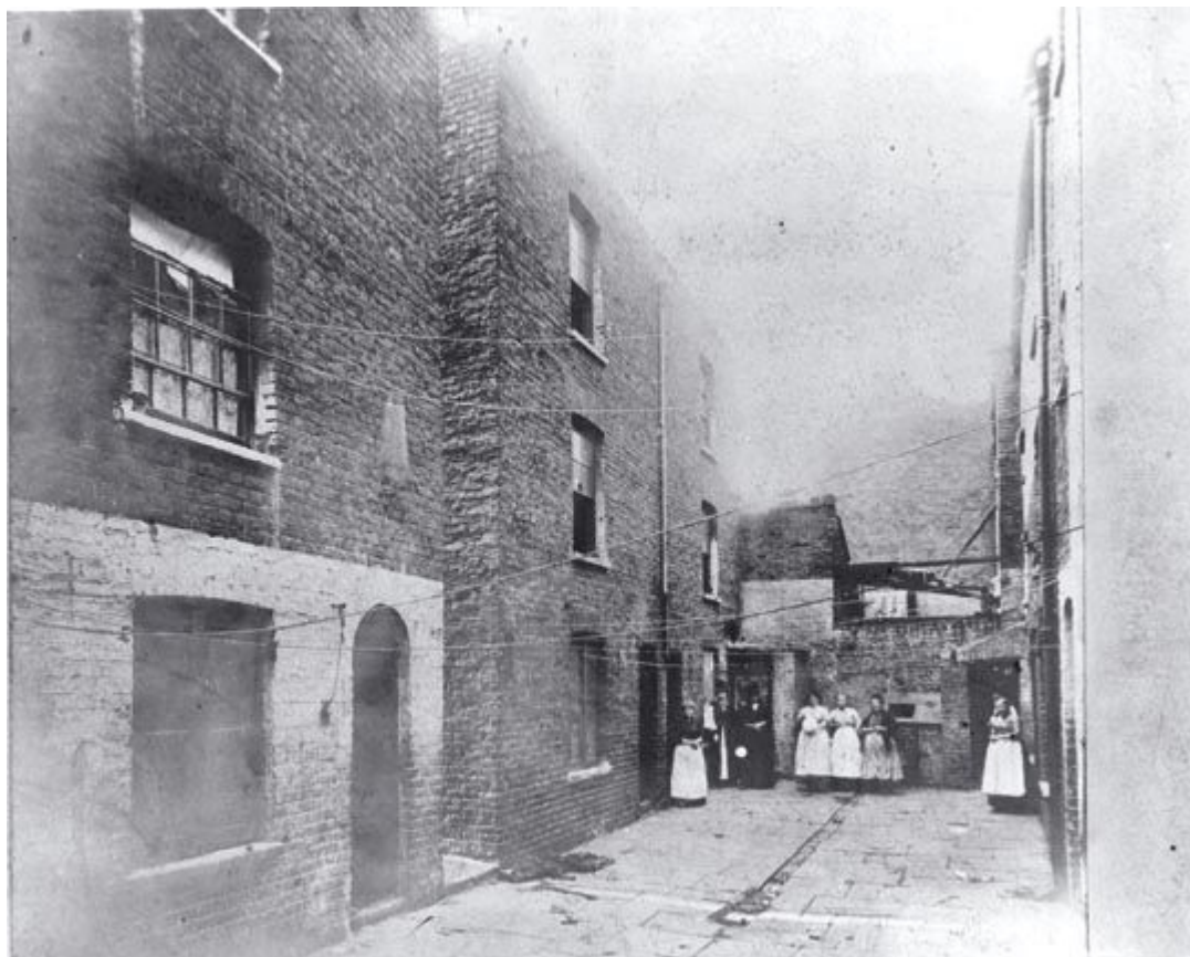
In Fr Jay's parish: a photograph taken off Boundary Street, Shoreditch, in 1890. Three years later, the London County Council began slum clearance, and the area was transformed into London's first council estate CITY OF LONDON METROPOLITAN ARCHIVES
